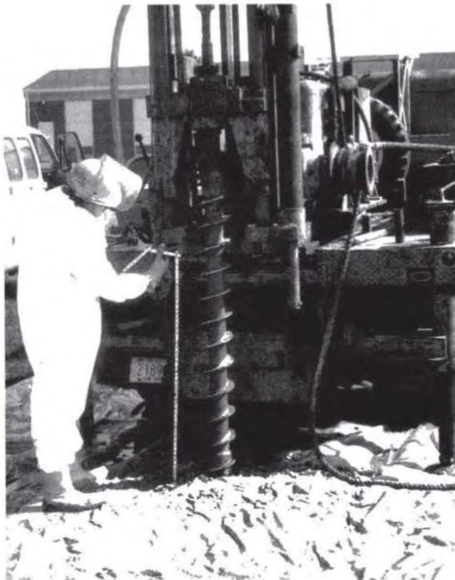
FIGURE 8.17 Hollow-stem auger drilling rig.
