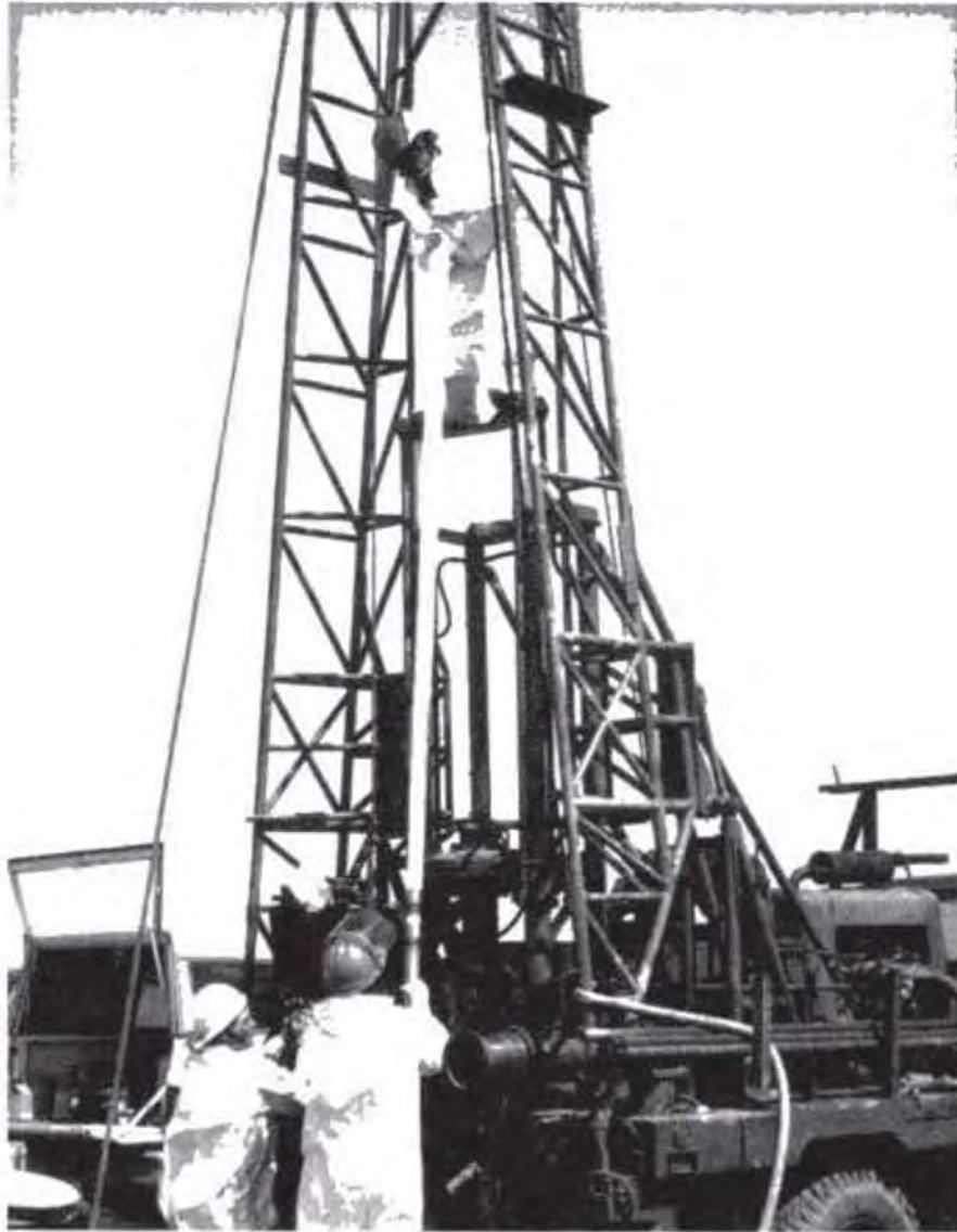
FIGURE 8.24 Lowering well screen and casing into hollow-stem augers. Note the white wrapping paper around the decontaminated casing.
